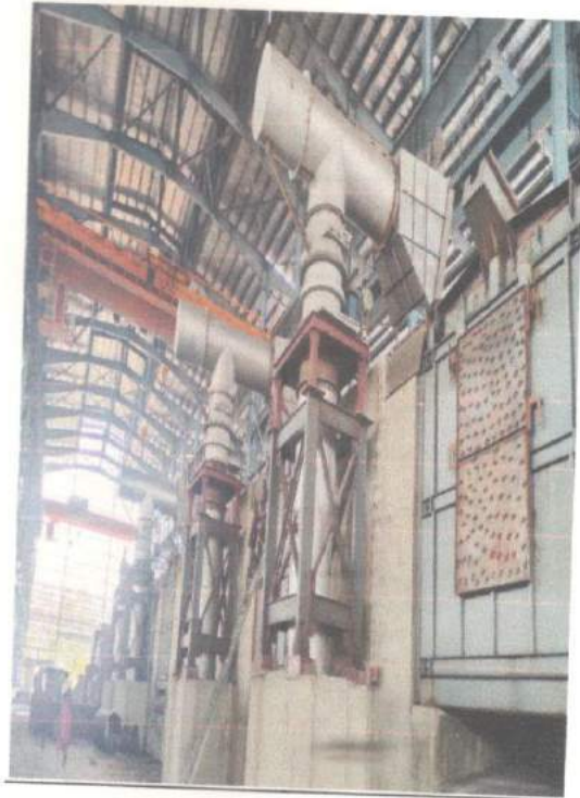
Bag Filter for Steel Smelting Shop
