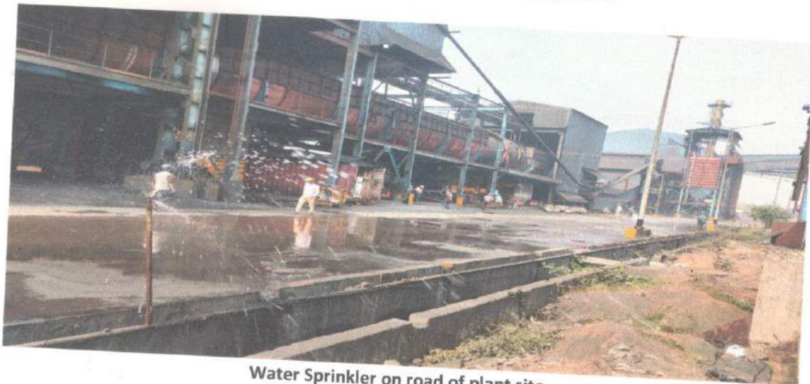
Water tanker for sprinkling on road of project site
