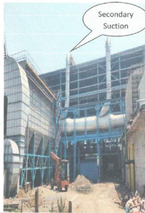
Primary & secondary suction connected with induction
